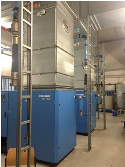
Compressor room Metal production ISRINGHAUSEN Lemgo
