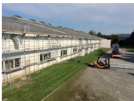
Roof renovation spring production Lieme (ISRINGHAUSEN)
