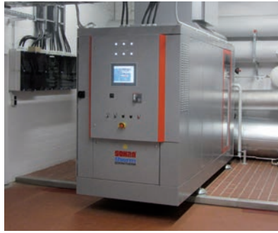
Combined heat power plant
